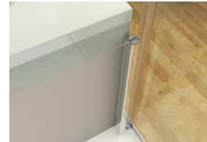
■ Details of the connection of shortened side wall to the bathtub
